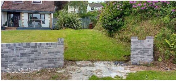
Driveway access from Leapmoor Drive
